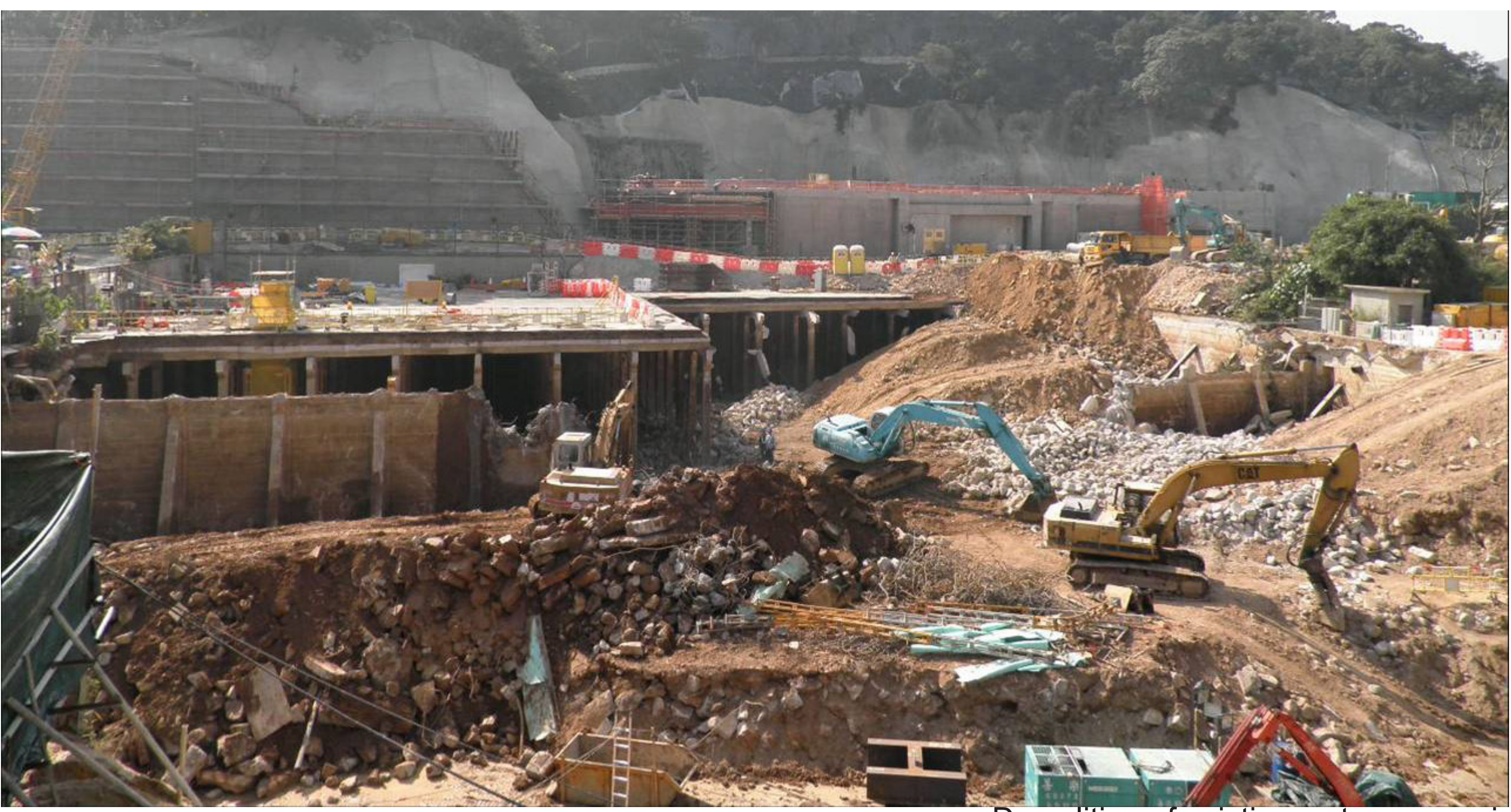
Demolition of existing water reservoir
